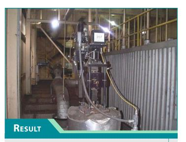
A supercritical plant operator will immediately notice smooth ramping startup valves that don't jump, stick, or overshoot. Putting a startup valve into auto mode for the first time is not uncommon. The ability to throttle bypass and level control valves at minimum travel becomes normal, thanks to 70mS deadtime, and a resolution of <0.1%.
