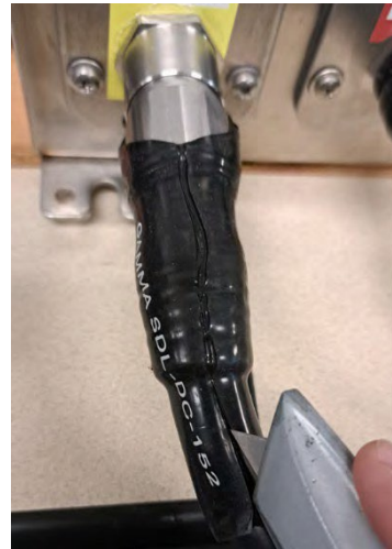
Figure 5B – Continue scoring all the way down to cable jacket to completely remove shrink
