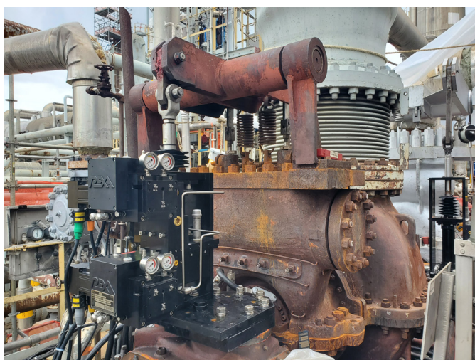
Figure 3. REXA before and after on a De Laval steam turbine.
