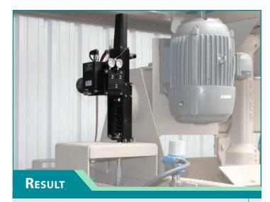
Upgrading from pneumatic actuators to REXA Electraulic™ Actuators on boiler feedwater recirculation valves can provide immediate benefits for any power plant. Maintenance savings can be immediately realized through tighter shut-off, improving trim life of the control valve, and reducing labor and material costs.
