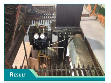
Always designed for "tough" modulating applications, REXA's Electraulic<sup>™</sup> Technology adapts to critical low duty cycle control for the TIV Bypass. The Electraulic<sup>™</sup> true closed loop hydraulic system is the difference to eliminate stubborn control issues, gain back reliability during startup, and assure reliable ongoing operations.
