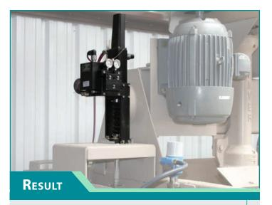
Upgrading from an oil pressure system to a REXA Electraulic<sup>™</sup> Actuator to operate wicket gates can provide immediate benefits for a hydroelectric plant. An upgrade to a REXA Electraulic<sup>™</sup> Actuator to operate wicket gates yield the following operational improvements:
