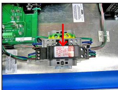
Photo 4.E.12.3-2 AC Power Surge Suppressor
