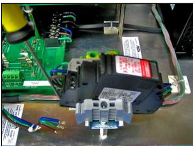
Photo 4.E.12.3-6 Release latch
