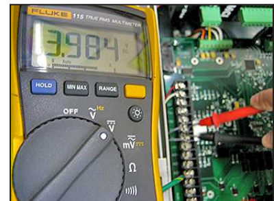
Photo 3.11-6 DC voltage for 20 mA
