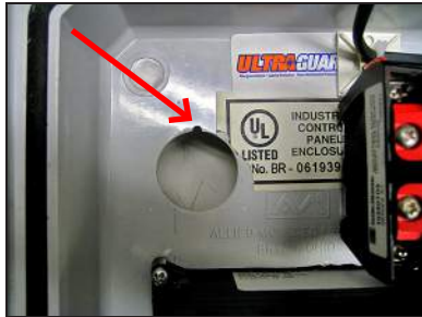
Photo 4.E.18.2-2 Notched enclosure hole
