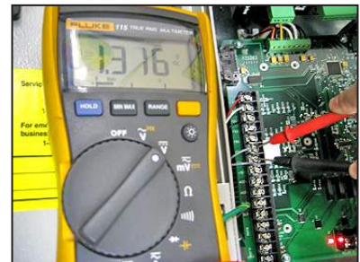
Photo 3.11-5 DC voltage for 4 mA
