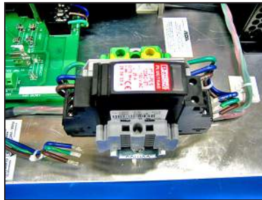
Photo 4.E.12.3-5 All power wires removed
