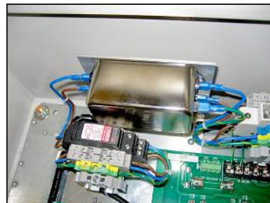
Photo 4.E.15.2-3 Complete Filter replacement
