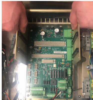
Figure 4.E.8.1-6 Interconnect Assembly Removal
